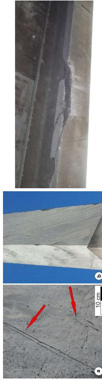
**Figure 1:** Two typical examples of structural health monitoring applications: left: non-destructive evaluation of the weathering state on a marble obelisk [14], right: typical damage of a bridge girder due to the impact of a truck [27].
