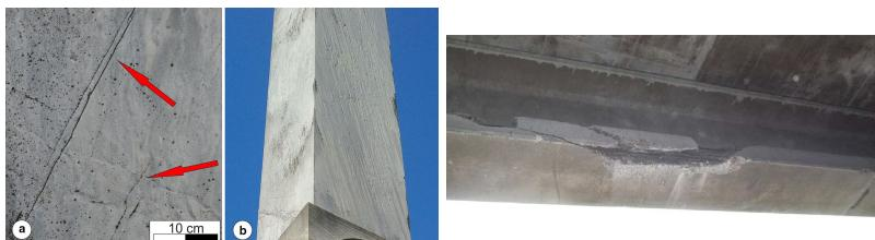
**Figure 1:** Two typical examples of structural heath monitoring applications: left: non-destructive evaluation of the weathering state on a marble obelisk [14], right: typical damage of a bridge girder due to the impact of a truck [27].
